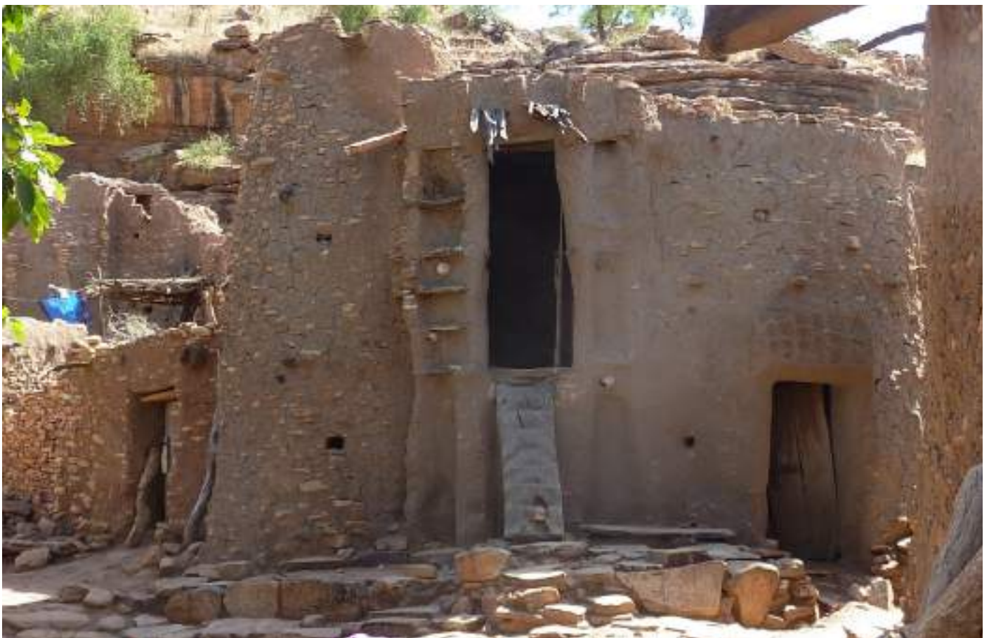
After the first step of renovation 2009
