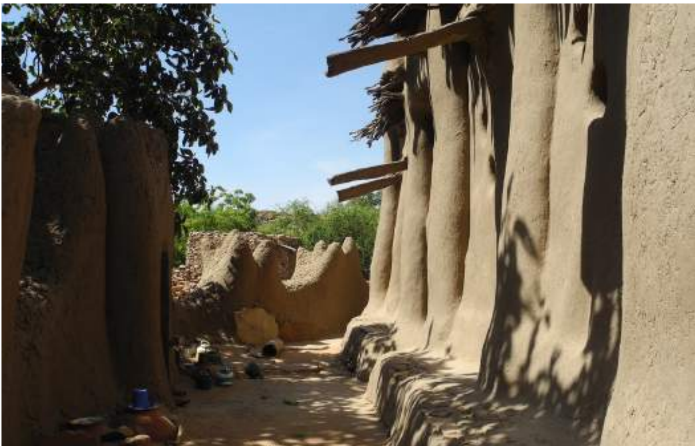
Details of the facades of the Mosque
