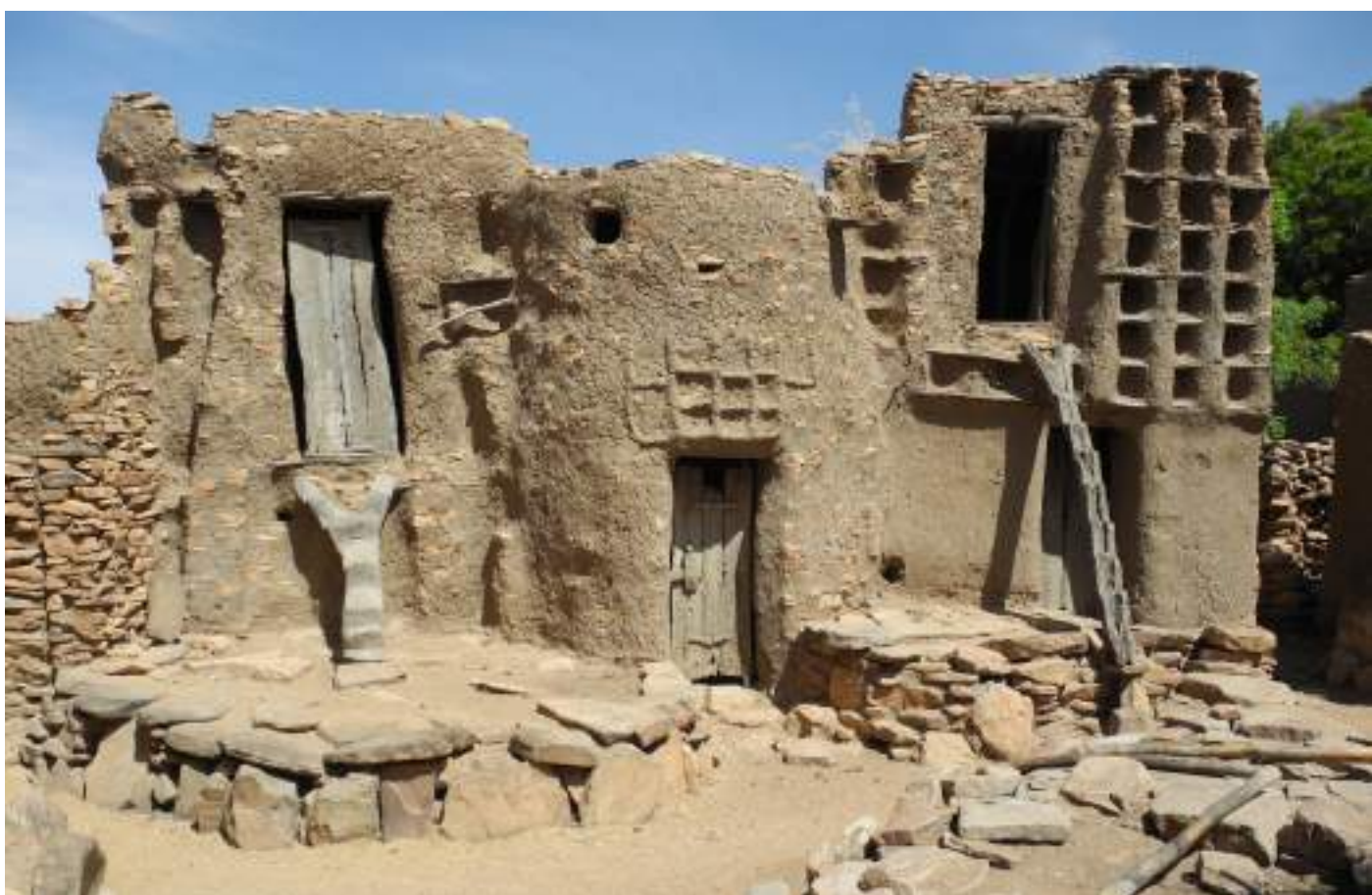
After the first step in the renovation 2009
