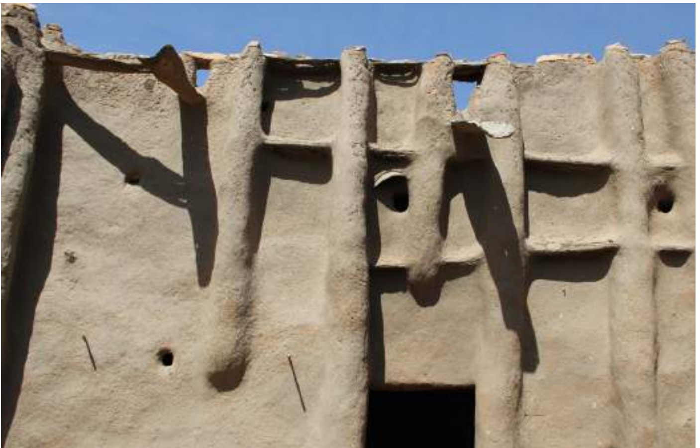
Detail of a family house 2020
