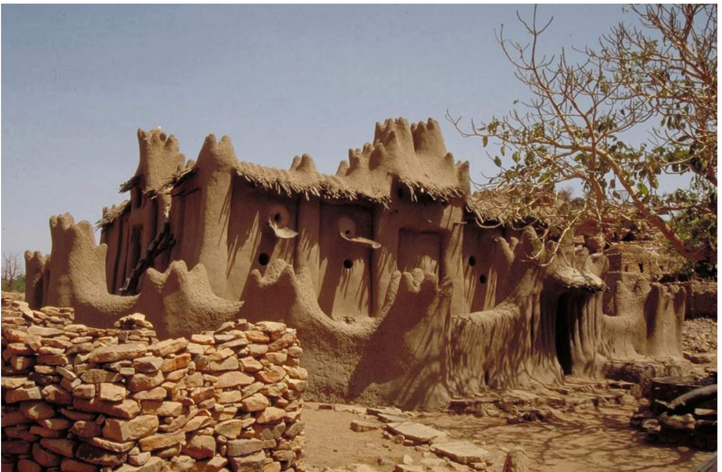
south east facade
