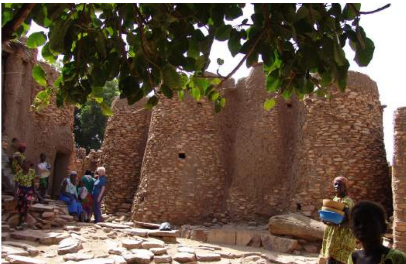
Family houses in 2002 still with some mud to keep the building construction together
