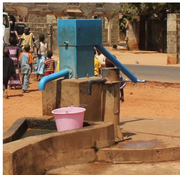
Another sustainable rehabilitated water point
