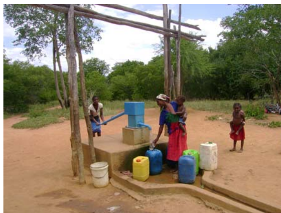
BluePump installed at 60m. in Mozambique
