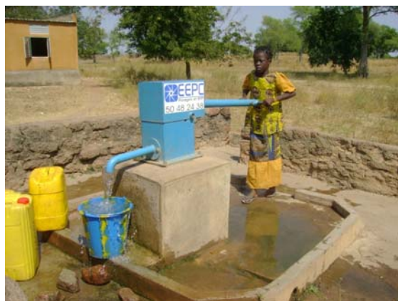
Bluepump on rehabilitated borehole, Burkina Faso
