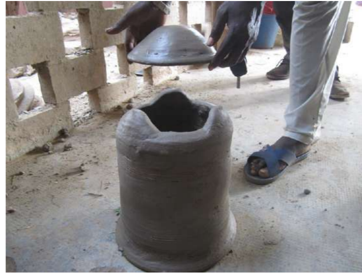
The handmade roof openings improving daylight and ventilation
