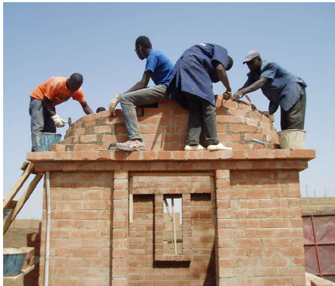
Internship of 10 students of the Technical School in Sévéré; the construction of the vault
