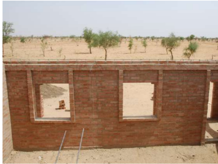
The wall openings of the classrooms
