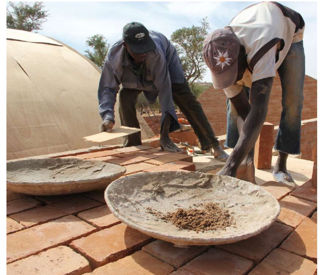
The construction process of a curved roof
