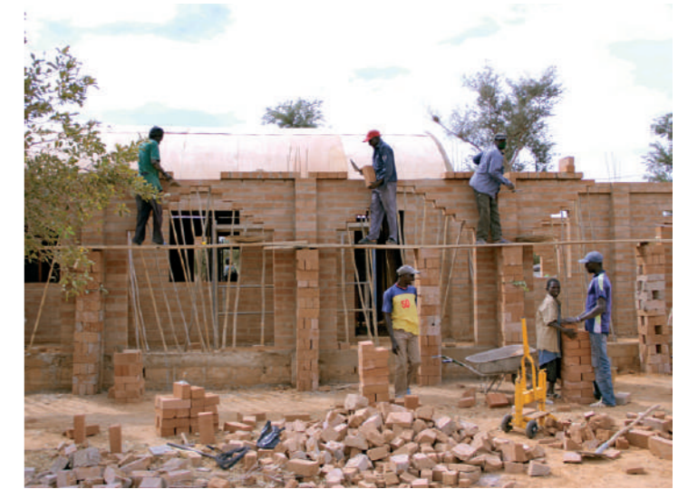
The roof is plastered
