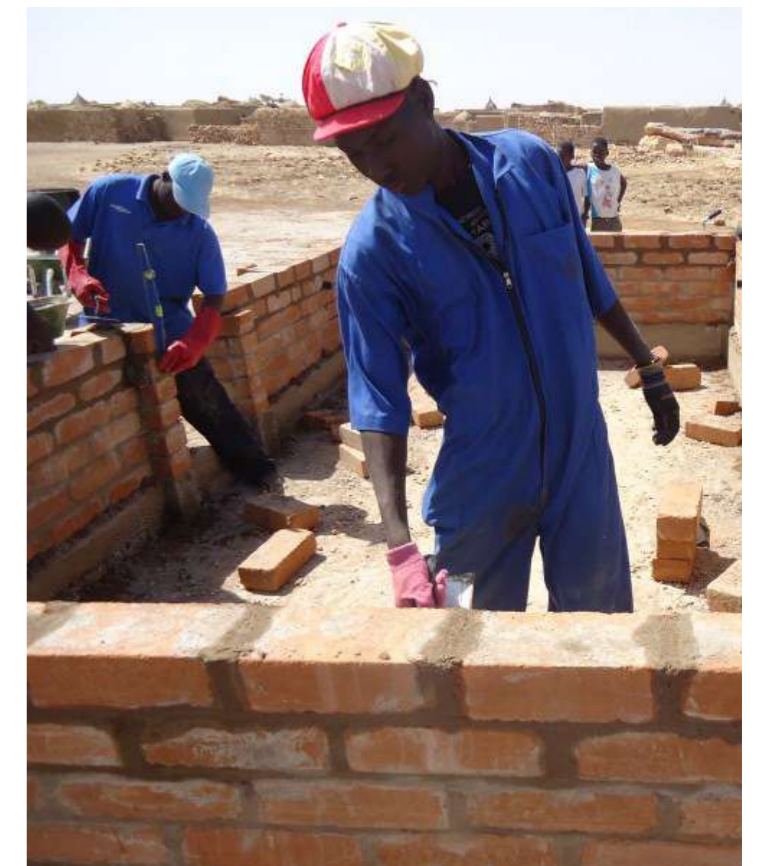
The construction of the wall with bricks
