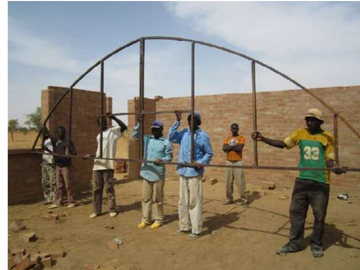
The steel frame functions as a part of the auxiliary structure
