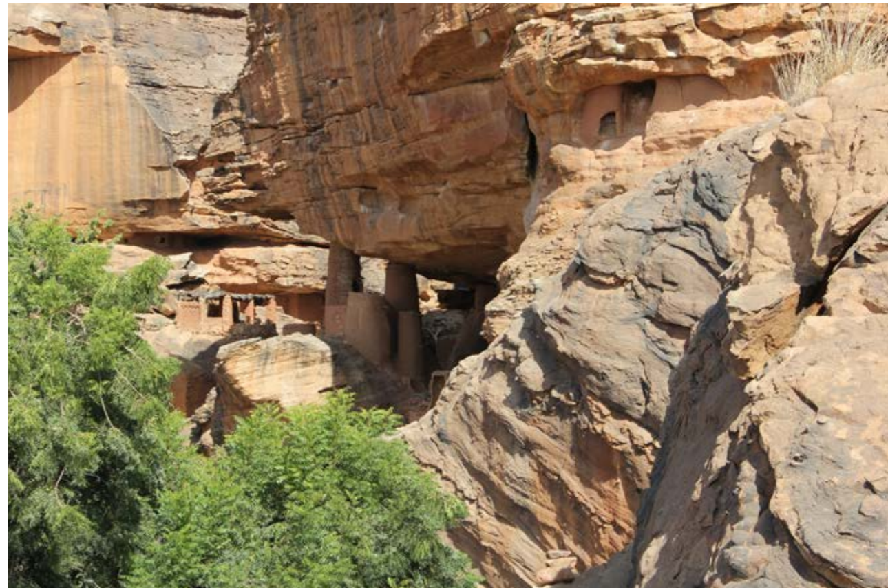
Situation Yougo Dogorou 2012, a few towers collapsed.
